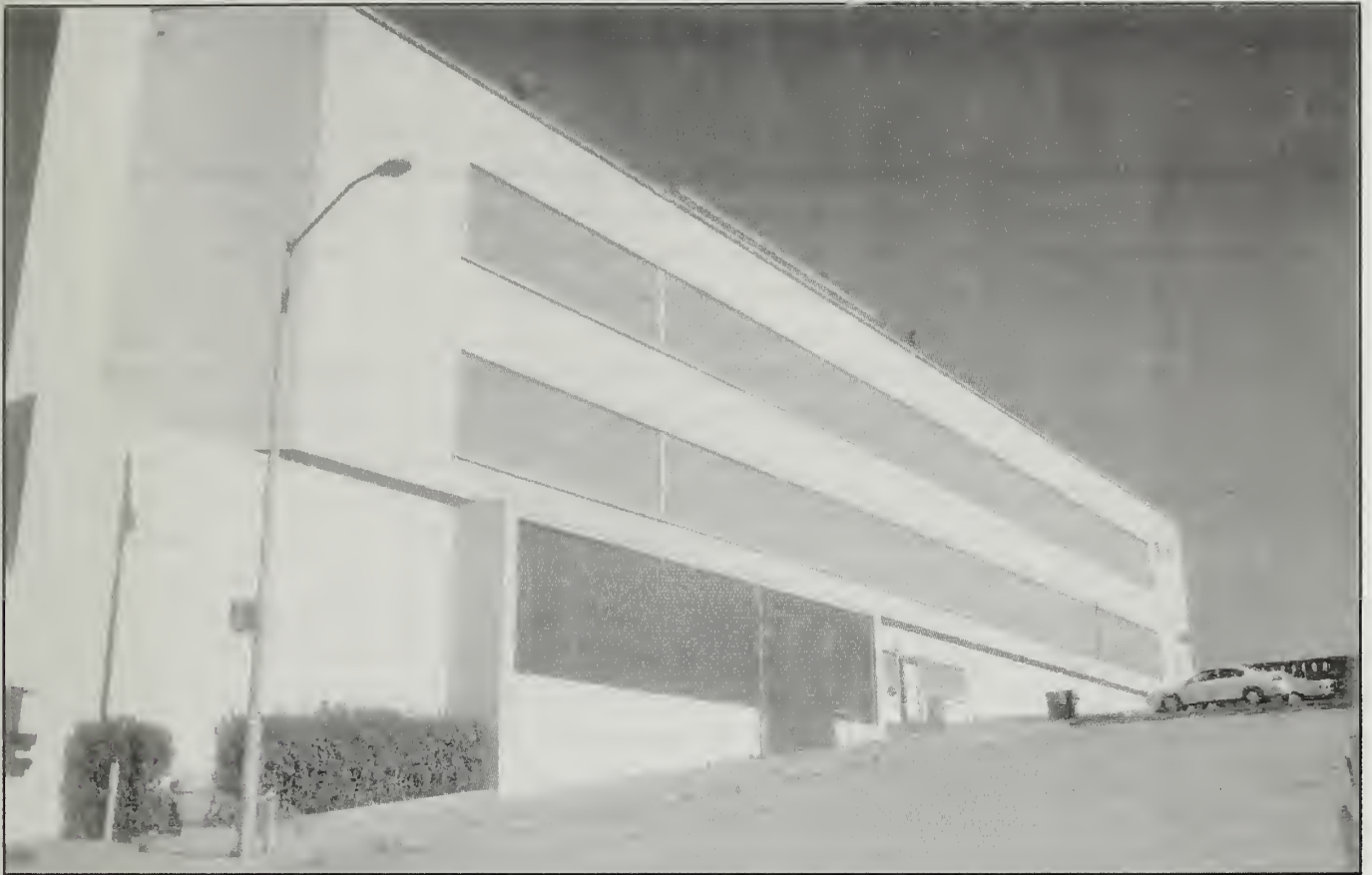
Figure 42 - Office Building, West Facade (First Street)
